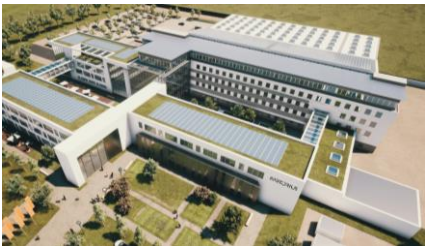
Expansion of bioreactor production capacities
