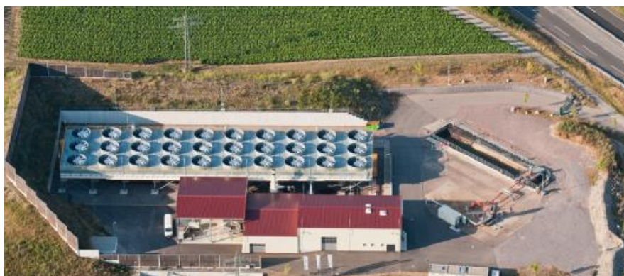
Picture: Geothermal power plant in Insheim, Upper Rhine Valley, Germany
